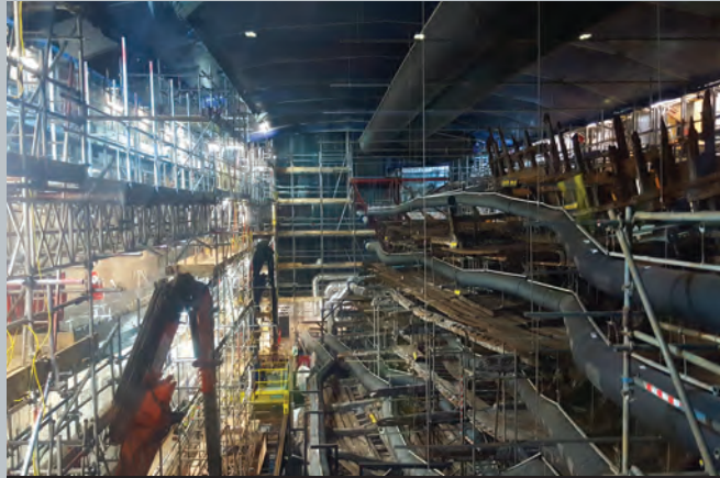
Ship shape: GKR used 150 tonnes of scaffold on Mary Rose
