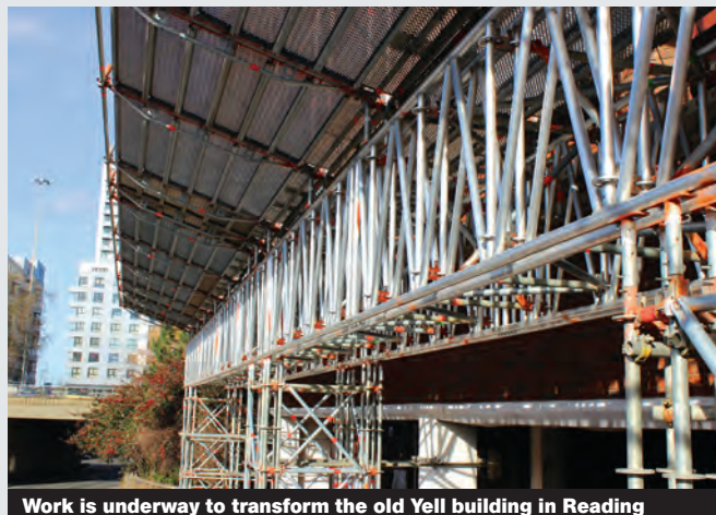
Work is underway to transform the old Yell building in Reading
