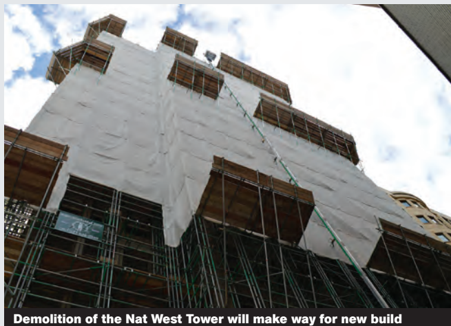
Demolition of the Nat West Tower will make way for new build
