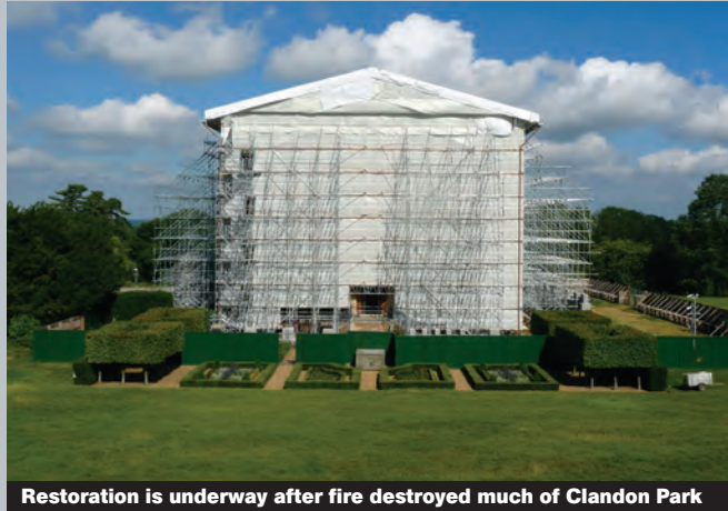
Restoration is underway after fire destroyed much of Clandon Park
