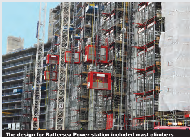
The design for Battersea Power station included mast climbers
