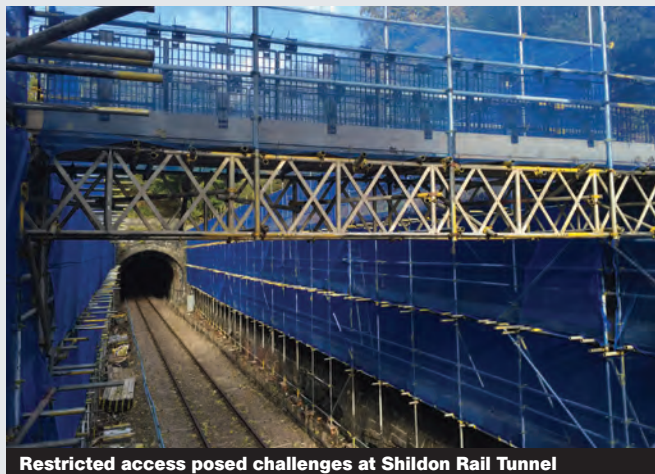
Restricted access posed challenges at Shildon Rail Tunnel
