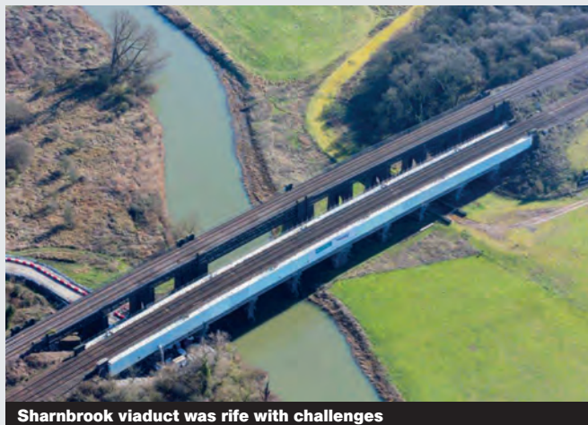
Sharnbrook viaduct was rife with challenges
