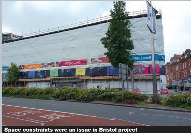
Space constraints were an issue in Bristol project
