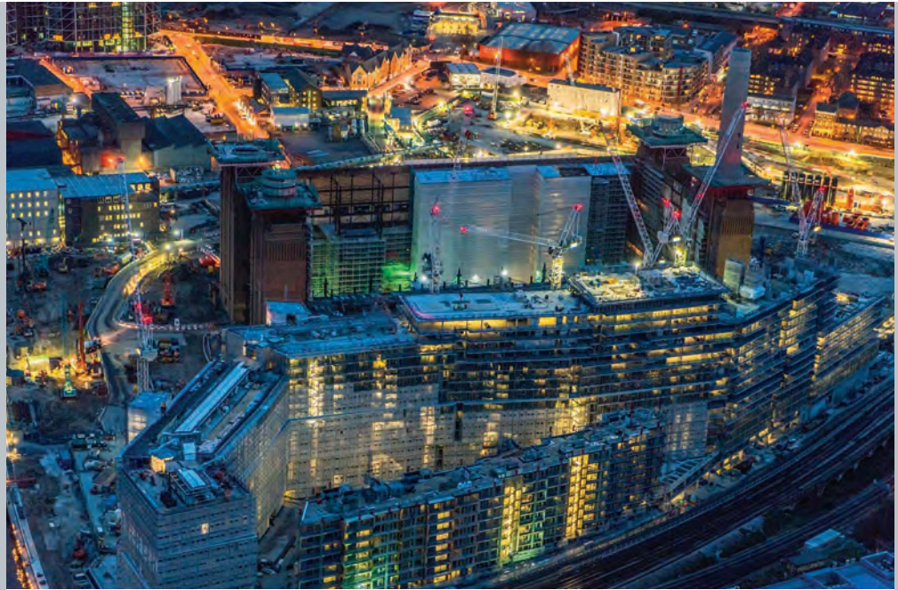
Erection of the 120,000m 3 birdcage scaffold on the East Wall Boiler House retention scheme.
