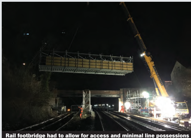
Rail footbridge had to allow for access and minimal line possessions
