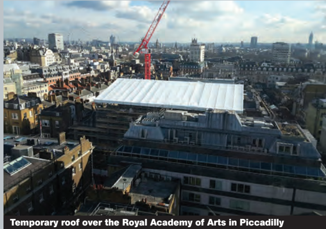
Temporary roof over the Royal Academy of Arts in Piccadilly
