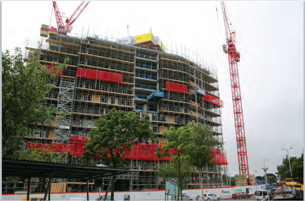
Beckley Court will be one of the highest building in the South West
