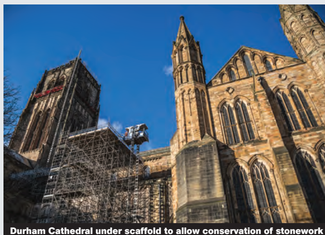
Durham Cathedral under scaffold to allow conservation of stonework
