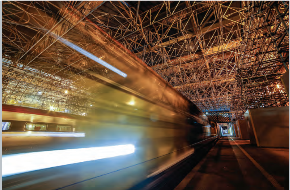
Carlisle train station currently features a bespoke scaffold system
