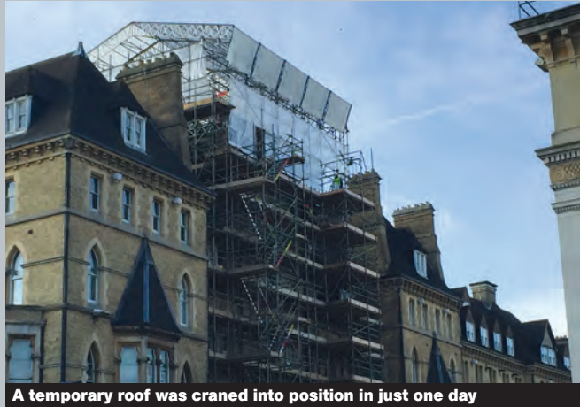
A temporary roof was craned into position in just one day
