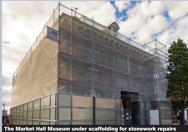
The Market Hall Museum under scaffolding for stonework repairs
