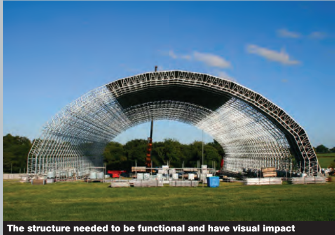
The structure needed to be functional and have visual impact
