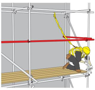
Figure 12: A scaffolder reaching below the single guardrail must be clipped on.
