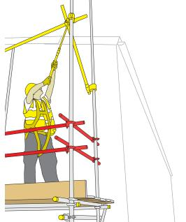
Figure 23: Push type Advanced Guardrail Tool (AGT) using special couplers and a positioning tool.
